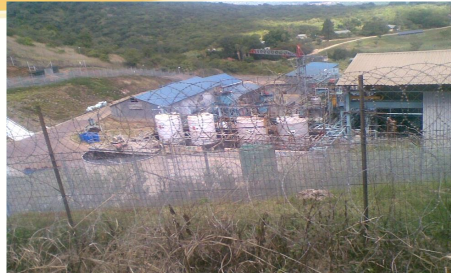
Fairview Bio Plant
